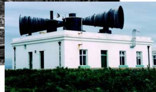
foghorns designed by Lord Rayleigh Trevoze Head Lighthouse, Cornwall (1913)
